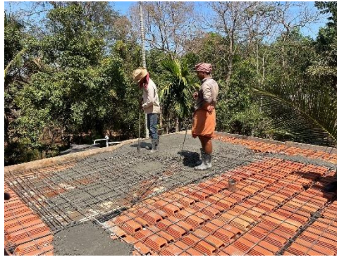
Fig.5: Preparation of Concrete
