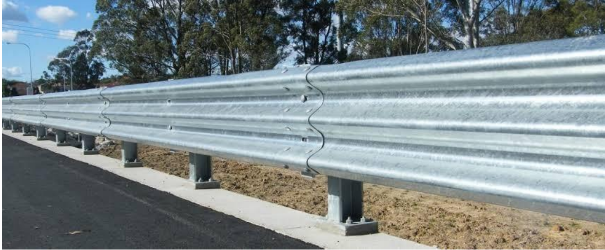
Figure 3: 1.7 Thrie Beam Steel Barrier (Source: www.alpharoofting.com )
