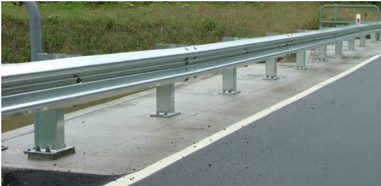
Figure 2: 1.6: W-Beam Steel Barrier (Source: www.dachugroup.com )
