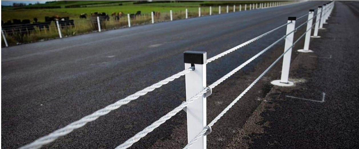
Figure 4: 1.8: Flexible Barrier (Source: www.Safe Direction.com )
