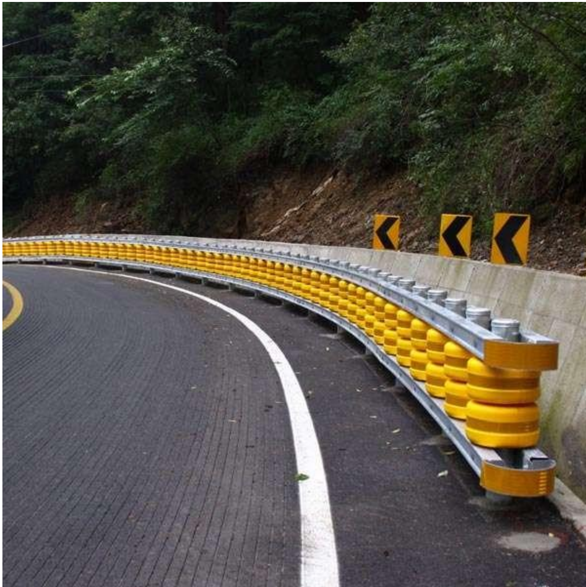
Figure 6: 1.10: Rolling Barrier (source: www.nikhilinfra.com )
