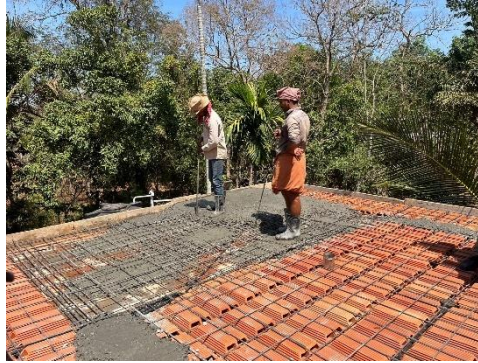
Fig.5: Preparation of Concrete
