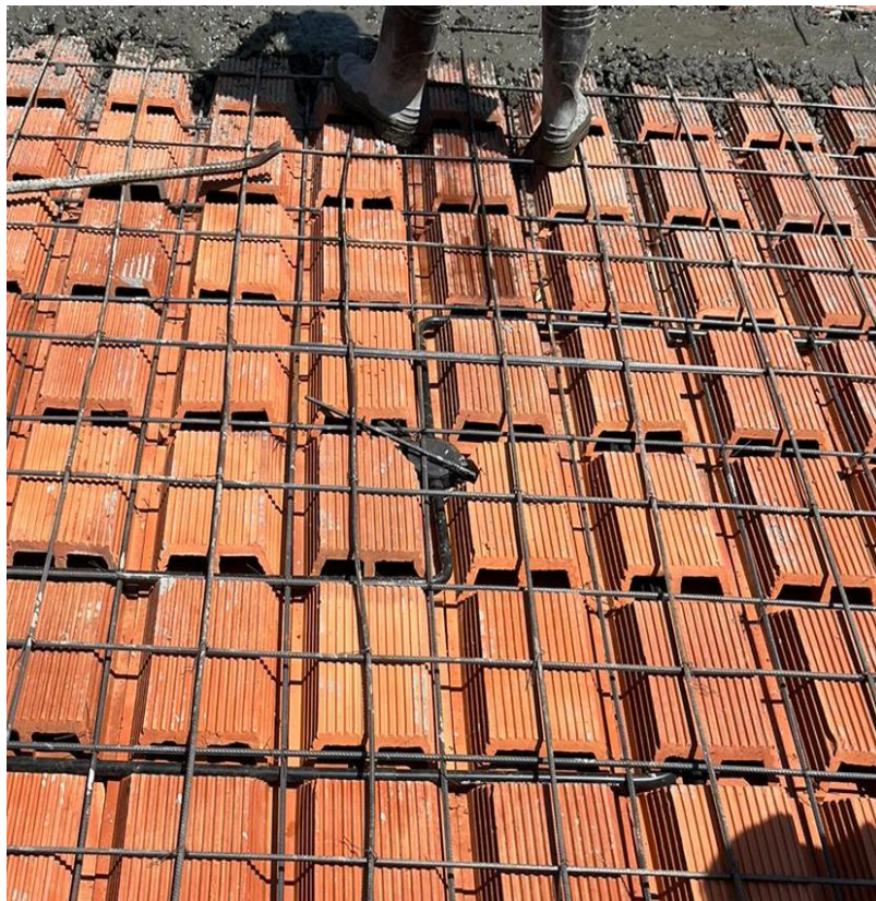
Fig.4: F. Concrete works
