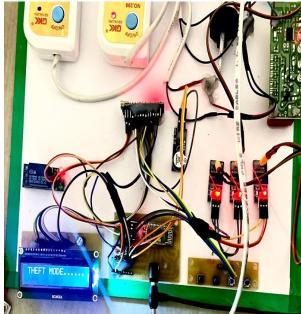
Fig. 2: Monitoring and analyzing electricity board-side energy
